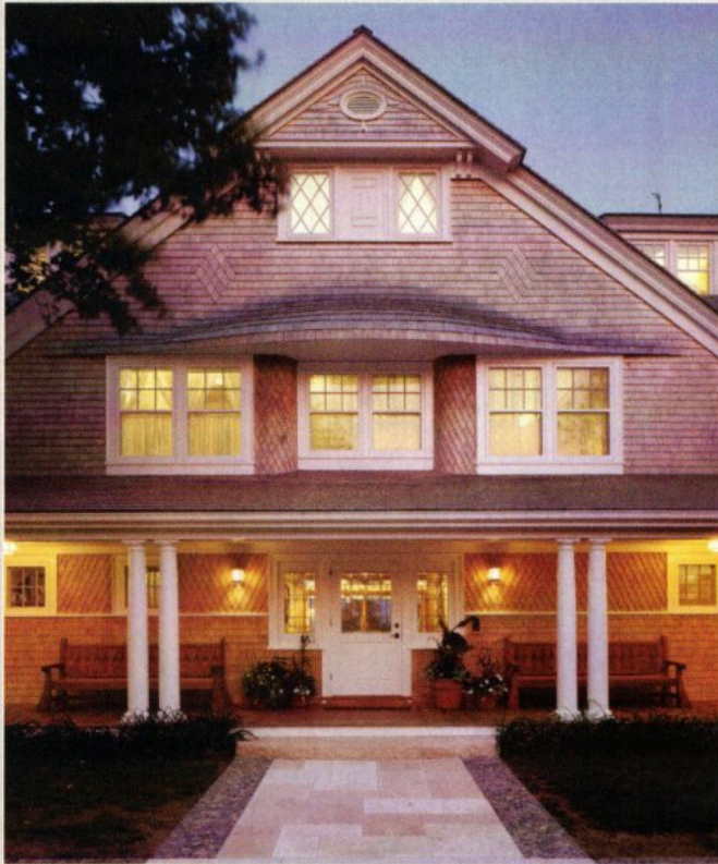
Brian Vanden Brink, Photography Mark Hutker & Associates, Architect
